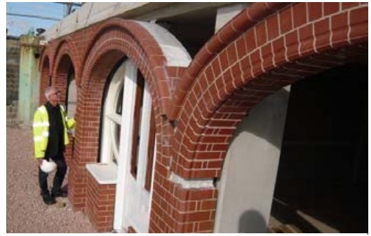
Cllr. Ian Davey, inspecting the new seafront arches during construction
